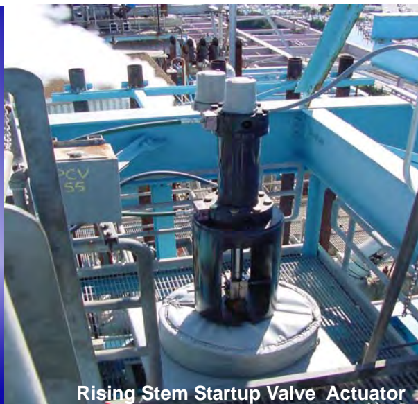
START-UP VALVE ACTUATOR
